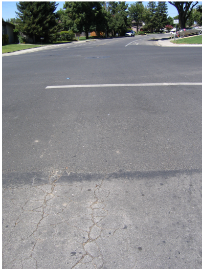
Figure 14: Overlay on El Dorado is doing well controlling the reflective cracks.
