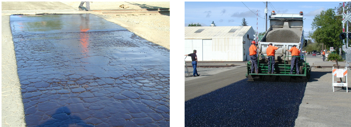
Figure 12: Left - PASS® emulsion penetrating the cracked original surface. Right - Application of the second layer of the double chip seal.
