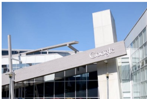
Unique and creative exterior signage is encouraged within the North and South Campus.
